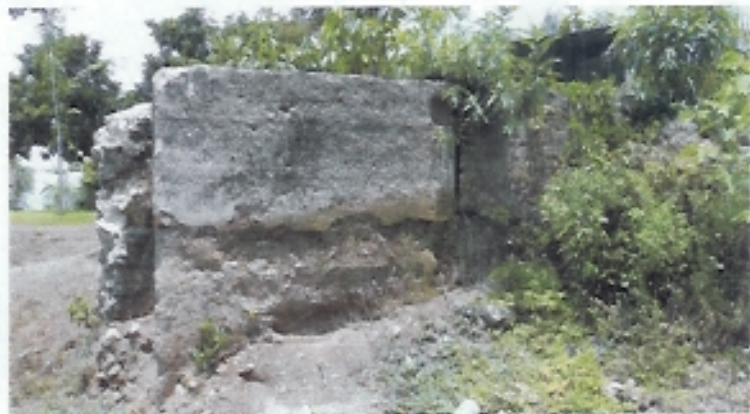
Plate 5 & 6. The adobe blocks with bricks used to fill in the gaps in the walls.
